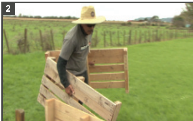
2 Cut pallets evenly in two halves.
