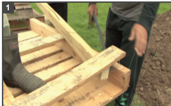
1 Remove back palings but keep intact to use again for capping.
